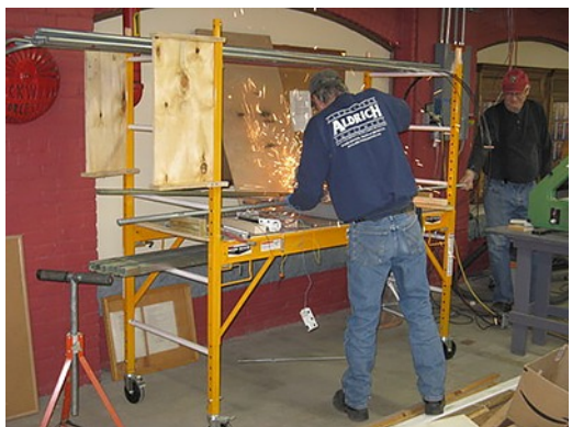
Sparks are flying as a member cuts conduit for the lighting circuits.
