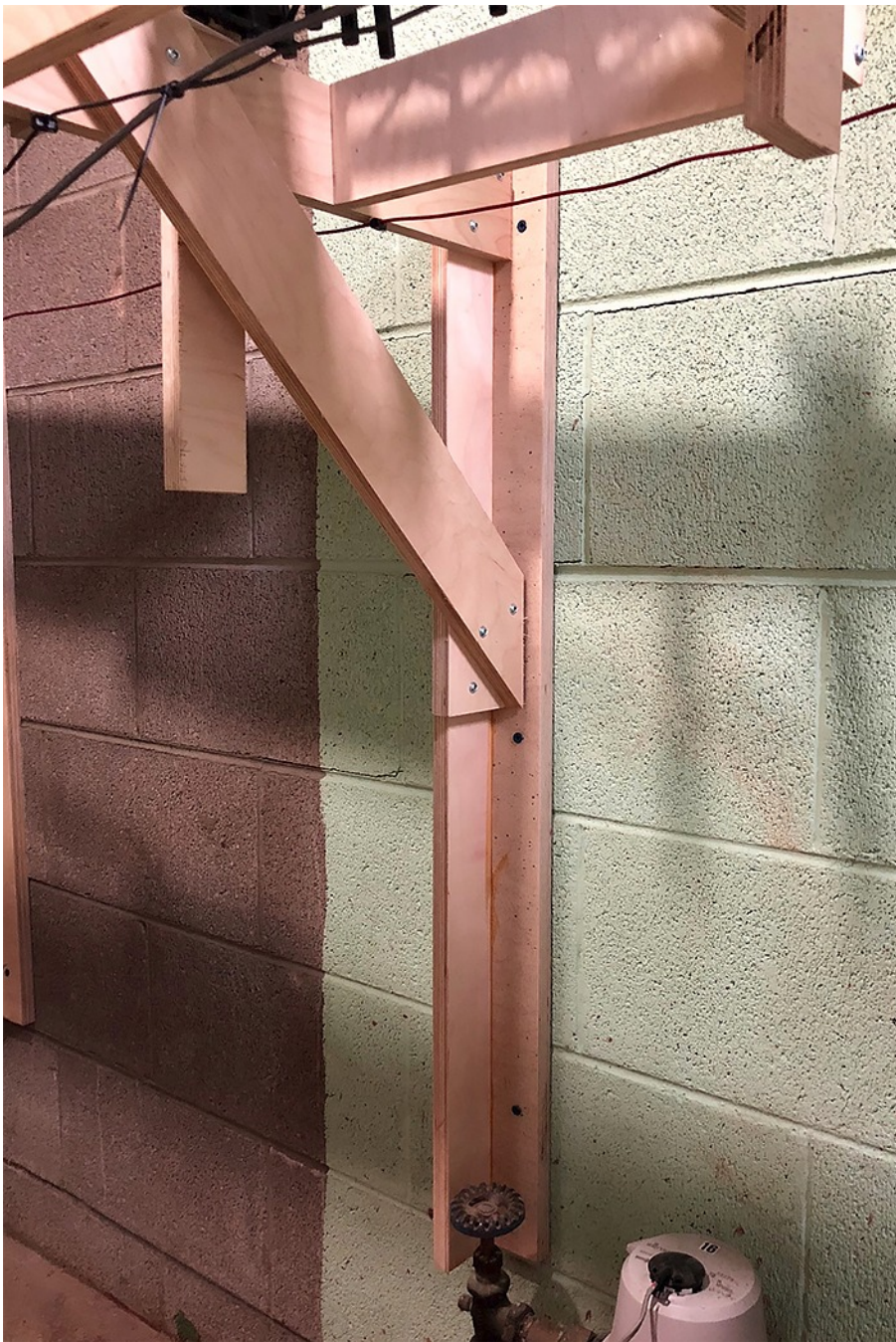
The bracket attached to the concrete wall. Note three, 1 3/4" concrete anchors spaced evenly. The benchwork is then built off of these brackets.
