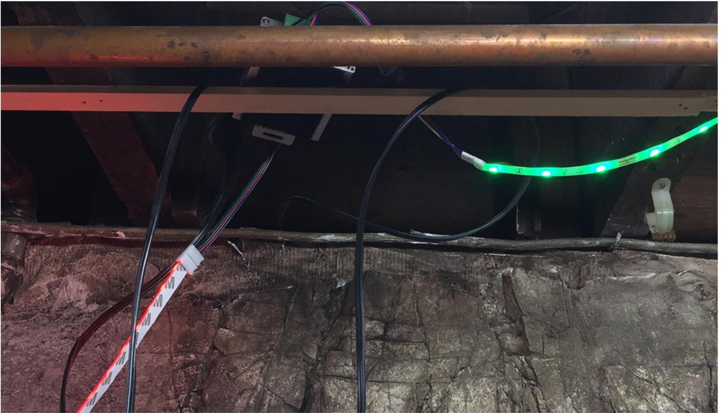
*And this is why we should bench test. Green on one string and red on the other. To fix, simply swap two wires (green and red) going into the amplifier and you are good to go.*
