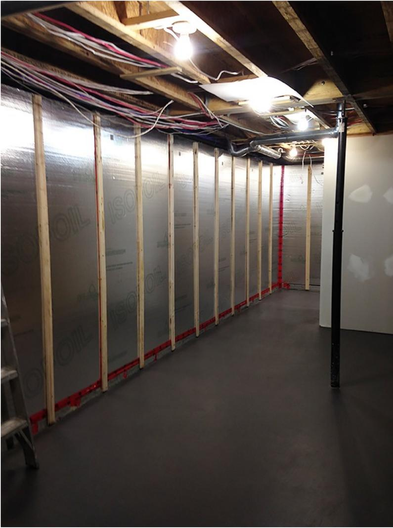
I then installed the lighting. I decided to go with standard light fixtures, as the cost would be much lower and this would allow me to pick and choose the type of lighting I want in the future. I installed 54 such fixtures lined up in the center of the aisles. For the moment, I am using 23 watt compact fluorescent bulbs. Perhaps when I get to the scenery stage, these lights will be replaced with something more color-friendly.
