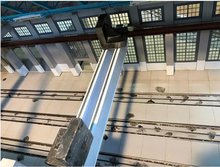
Gravity clamps held the gantry tightly to the trucks until the epoxy cured keeping the assembly aligned.
