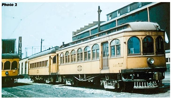
An extra high knuckle was important for some systems to avoid parting the train on severe vertical curves where the tracks were in the roads. These high knuckles led to the development of similar couplers for steam road use particularly on tank cars to reduce the likelihood of couplers parting during derailments. When steam road cars parted, there was the danger of one coupler piercing the end of the adjacent tank resulting in spills, fires and/or explosions.
