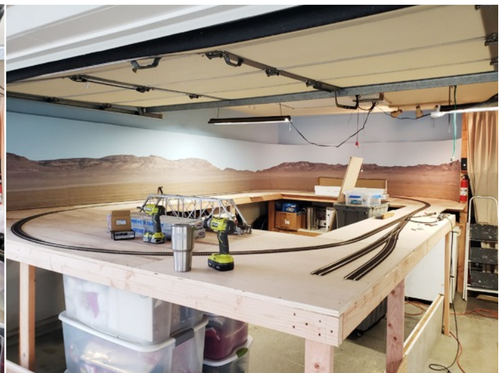
Layout under construction.
