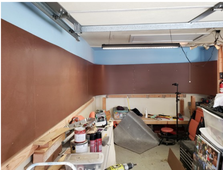
Here is the layout under construction before the backdrop was installed.
