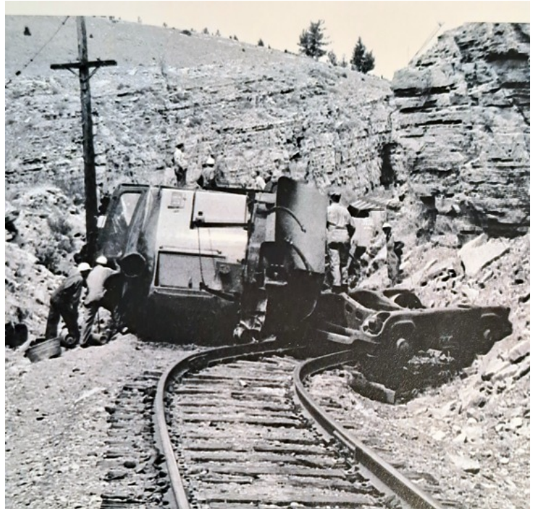
The amount of force in play here was quite obvious. 300 tons of steel lays on its side.
