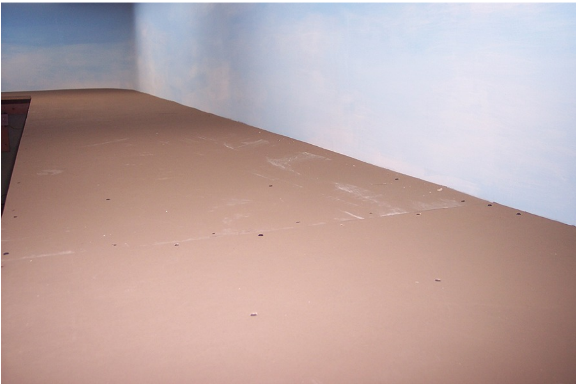
The top picture shows the plywood sheets for the decking with the storage underneath. Next, the Homasote was glued and screwed to the top, being careful to overlap the plywood seams.
