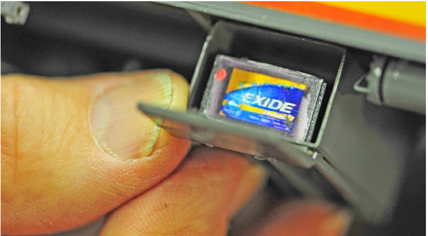
The battery box on this Milwaukee Road car even has batteries in it with a working lid on the box.
