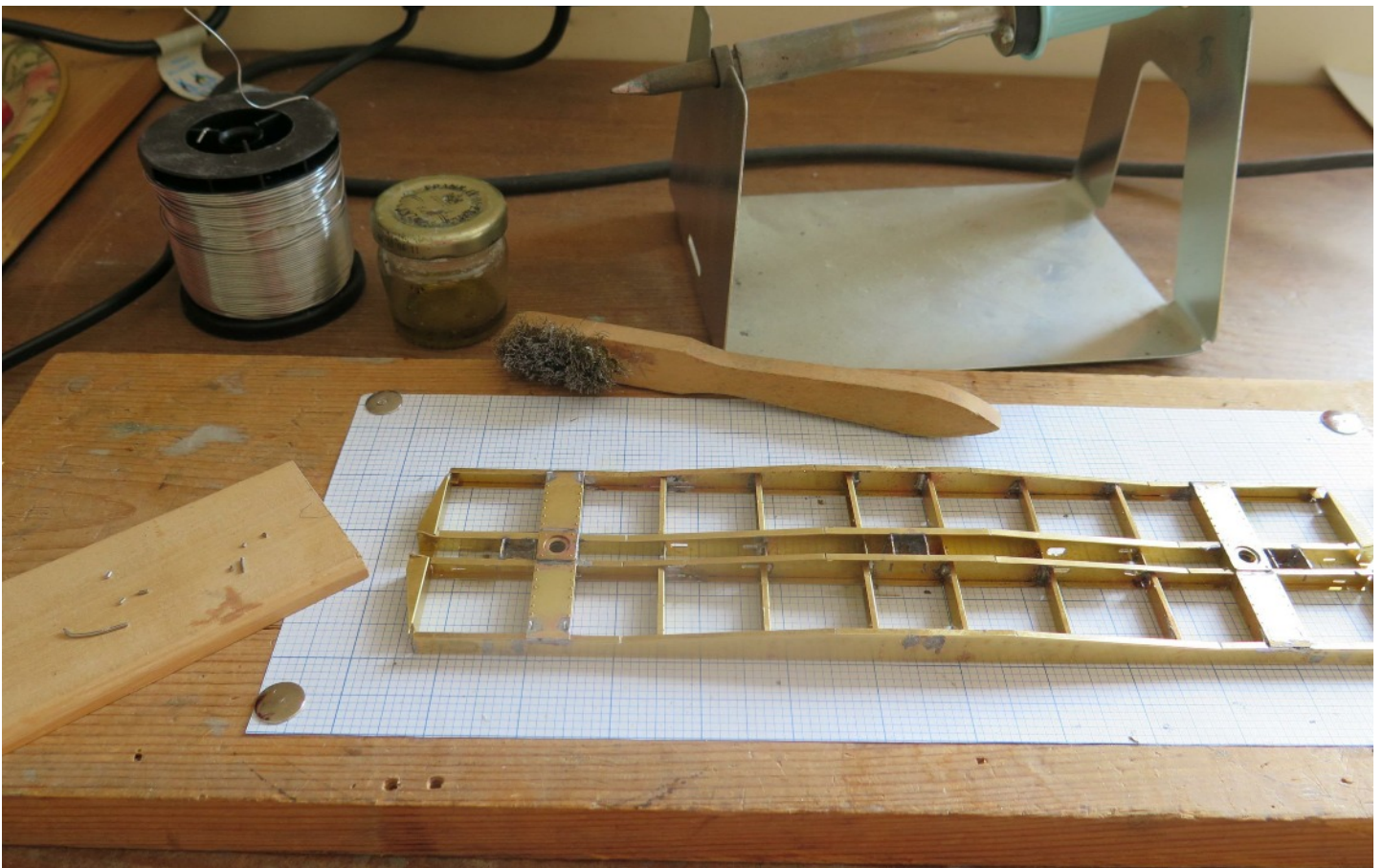
In order to make sure the frame was assembled square, Tim built it on a piece of ruled graph paper. Once you get a few of the joints made, they will hold the frame and you can remove it for more soldering. Keep checking as you go.
