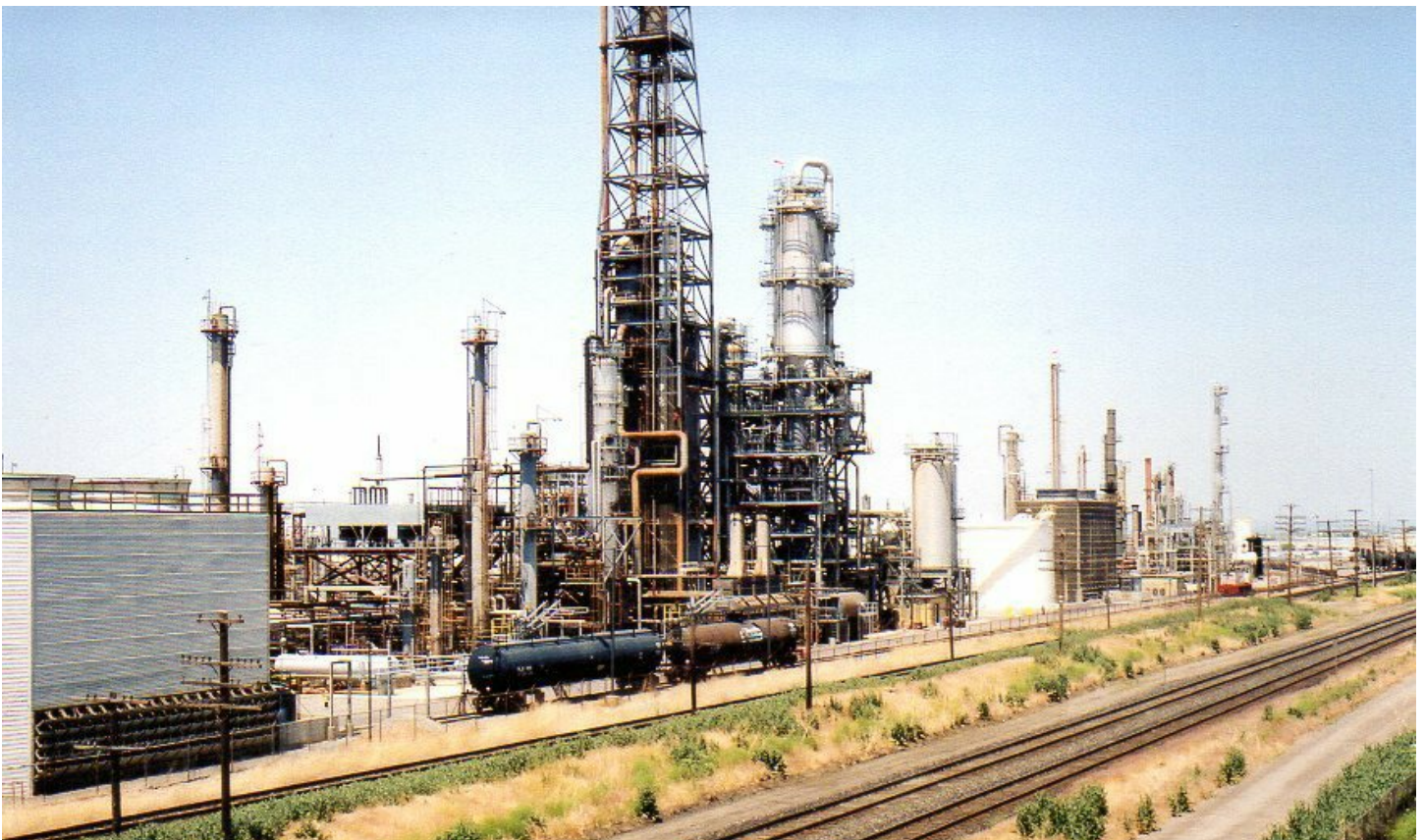
There is a refinery in Ogden, Utah, and Bill took photos of it on his trips to the area so he could make a model on his layout. The bottom photo is one of the photos he took. A friend of Bill's works in refineries and helped him get some of the details right and explain what all the piping was for. Bill's model, while quite compressed, captures the feel of a refinery. Less size and more detail usually works.
